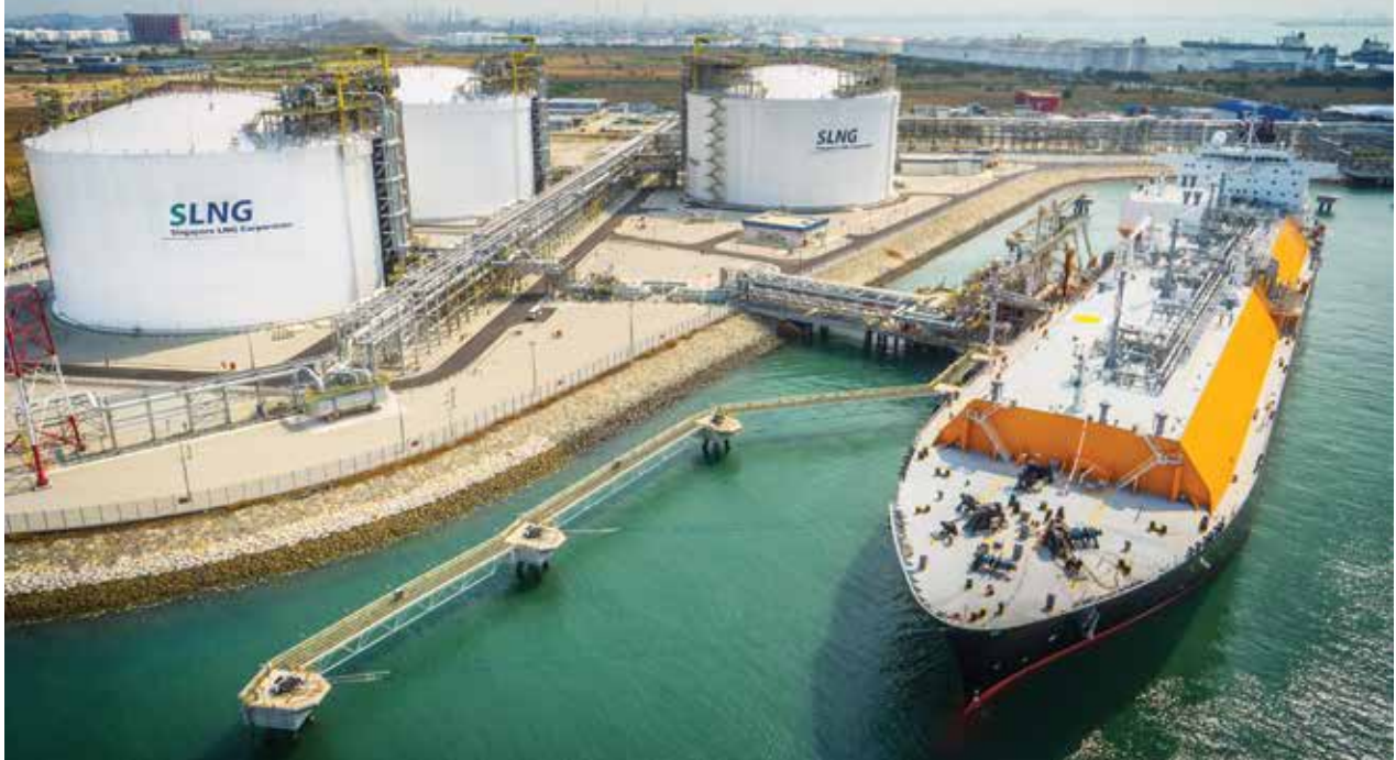
Liquefied Natural Gas (LNG) Terminal on Jurong Island
