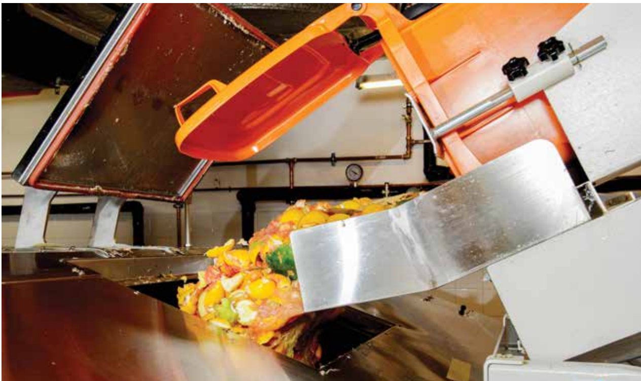
In-situ food waste recycling at Marina Bay Sands
