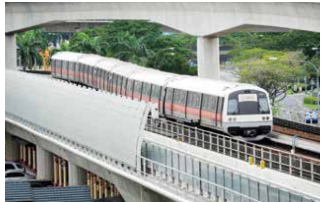
Noise barriers near Jurong East MRT Station
