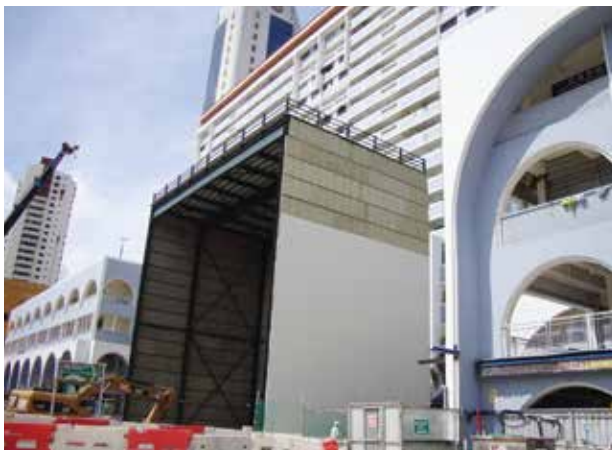
Noise barriers being used in an LTA construction project
